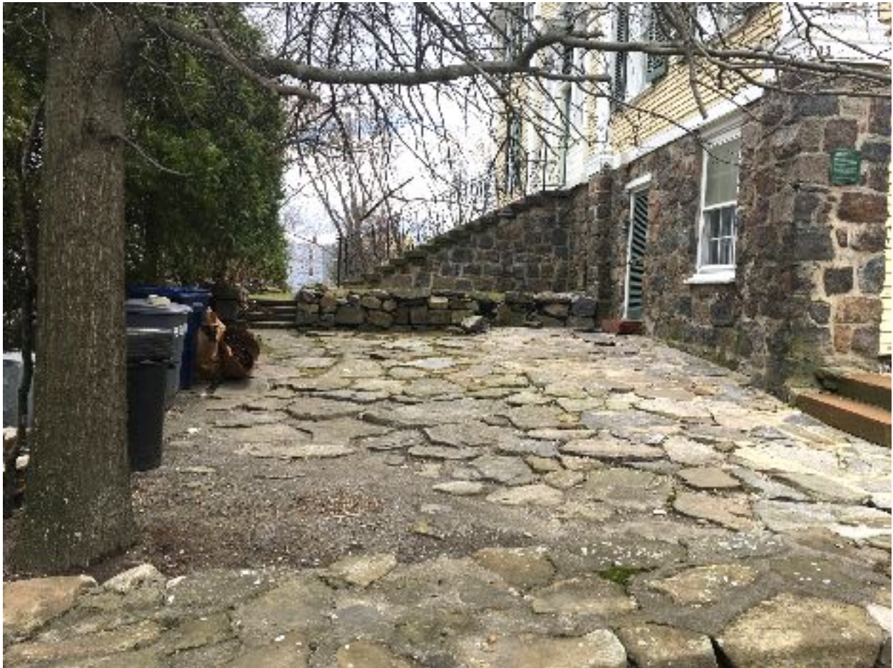
Figure 4- Stone landscape and stone retaining wall (in front of steps) on northwest side of House to be improved after archaeology. View facing east. Original 1747 foundation expected in this area. Note stone from retaining wall (and possible privy) dislodged and currently sitting on paved area.
