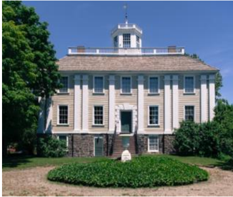
The Mansion's major exterior paint and wood repair project was completed in the fall. Shown here in July before shutters were re-hung, the Georgian pilasters appear even more prominent. Photo: Bill Finch
